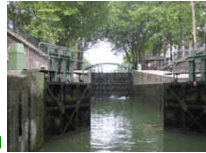
[ The lock gate in Canal St-Martin ]
