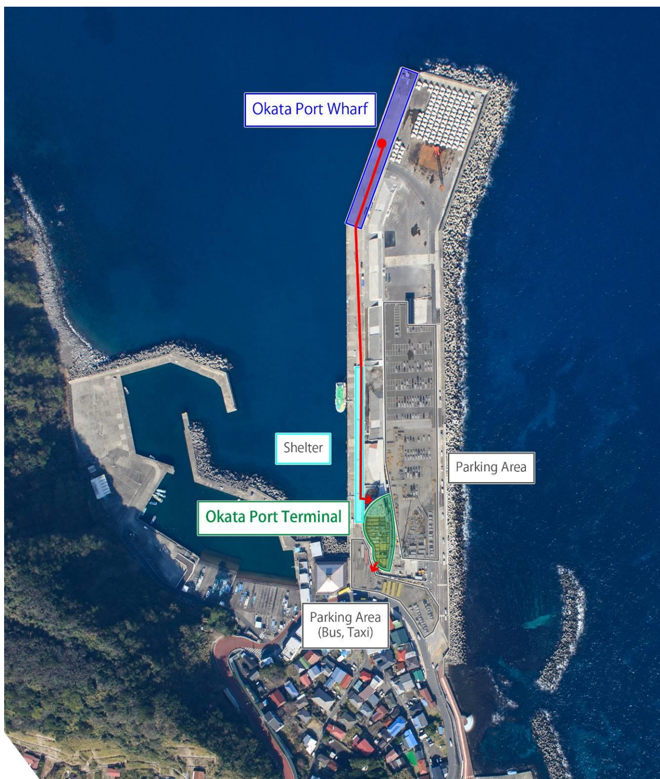
Figure of the terminal placement and passenger line of flow ターミナル配置図と受入動線
