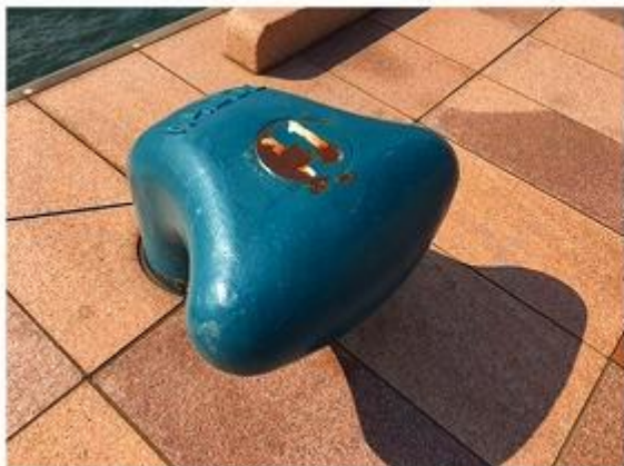
Bollard 70t 20m interval 11.
