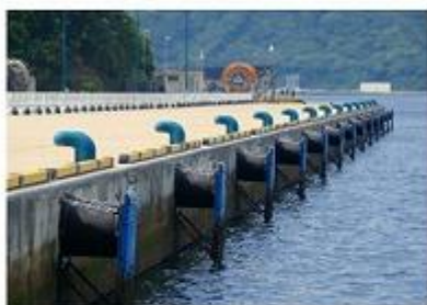
Fender 20m interval 13.
